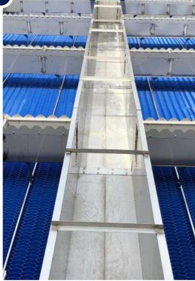
The design and arrangement of the effluent launders has an impact on the overall settler performance.
